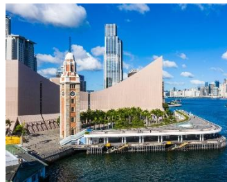
TST Clock Tower
